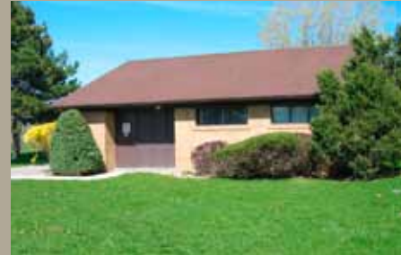
Substation House Scarborough
