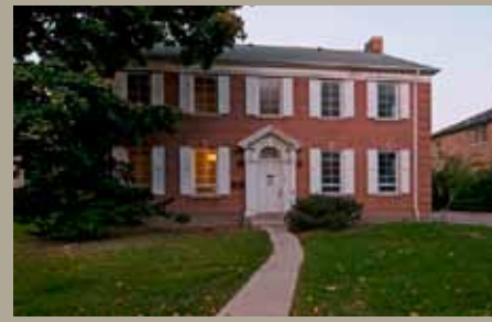
Substation House 555 Spadina Road
