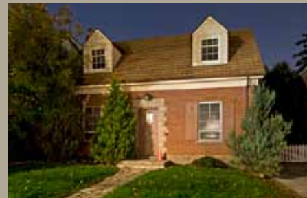
Substation House 640 Millwood Road
