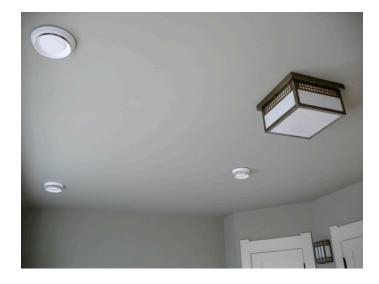
Figure 13 - HRV supply vents, located on the ceiling of the second floor master bedroom
