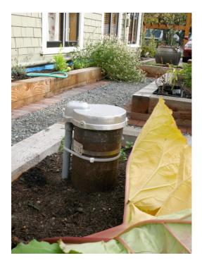
Figure 14 - Geothermal well head (disguised by raised vegetable bed in south side garden)
