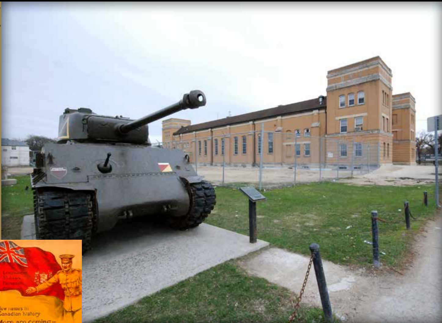
Above and right: McGregor Armoury, 551 Machray Avenue, Winnipeg, has been part of the St. John's neighbourhood since its completion in 1914.
