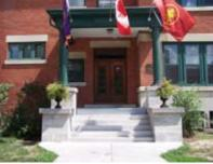
The steps themselves were dismantled and replaced with five new quarried limestone slabs, cut and hand finished to replicate the original bush-hammered appearance of the steps. The end result is a welcome improvement both visually and in terms of safety!
