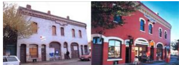
Hart Block, 529 Herald St. before and after its rehabilitation. Credit: Steve Barber, City of Victoria (before) and John C. Taylor (after)
