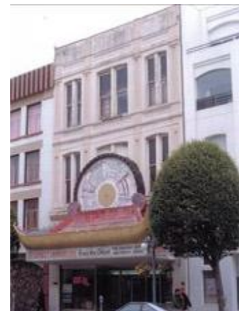
Royal Victoria Suites, 1411 Government St. before restoration work. Credit: Steve Barber, City of Victoria.
