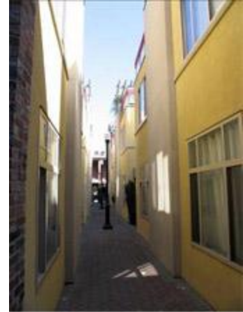
The "Dragon Alley" project involved the adaptive re use of Chinese tenement buildings from 1912 which had been vacant for over 20 years. The alley is now a pedestrian pathway that allows additional light into the residential units.
