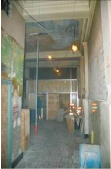
Interior of Lougheed Building before its restoration
