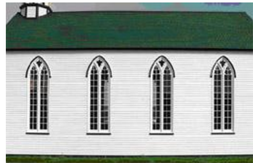
Restored windows, St. Joseph's Catholic Church, Bonavista. Credit: Brian Ricks
