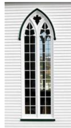
Restored window, St. Joseph's Catholic Church, Bonavista Credit: Brian Ricks
