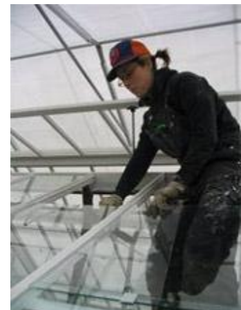
Hoff Boyle completes glazing the south side of section five
