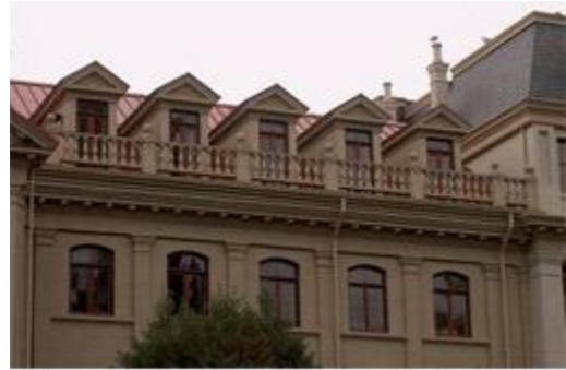
Restored dormer windows at St. Ann's Academy, Victoria
