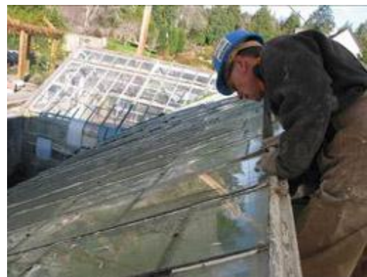
Davyd McMinn begins removing glass from section four of the greenhouse
