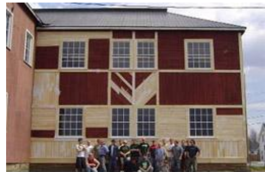
Restored Agricultural Hall, 2004
