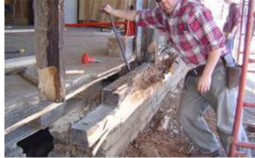
Restoration of the Almonte Agricultural Hall, 2004
