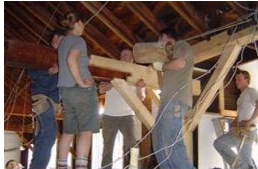
Restoration of the Almonte Agricultural Hall, 2004
